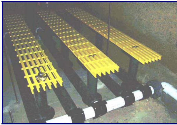
(a) Installing diffusers and assembling piers and grating as media supports
