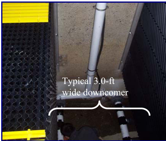
Figure 5 Downcomer region showing access to diffuser manifolds
