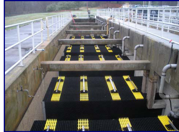
(d) Overview on the completed media towers
